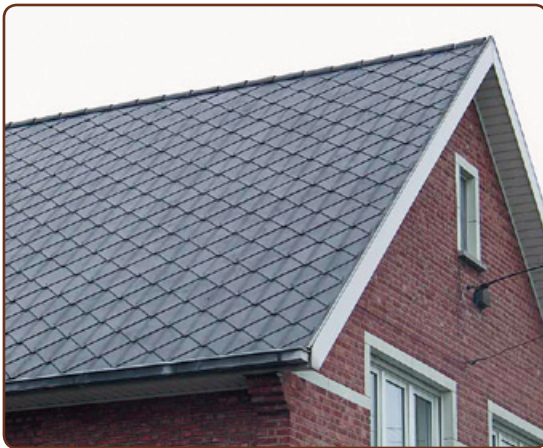
Dakleien in asbestcement
